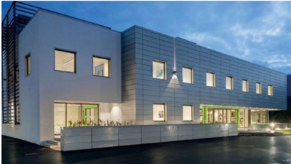
AAA's headquarters in Saint-Gents-Pouilly, France, just across the border from CERN. Image credit: AAA.
